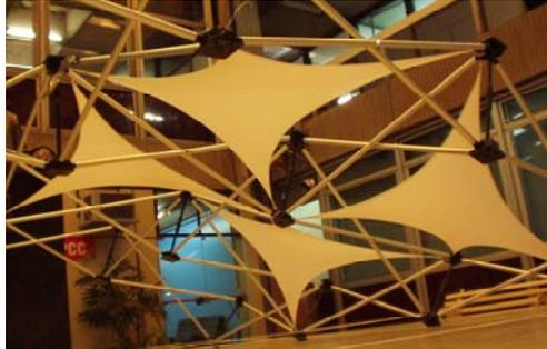
Figure 6. Membrane application to pantographic structures by Titti Titotto, 2003
